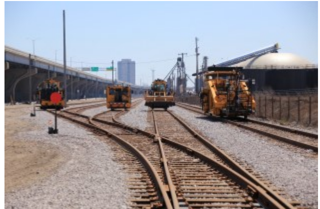
New Yard tracks at Milwaukee Harbor April 17, 2016. Photo by Keith Schmidt
